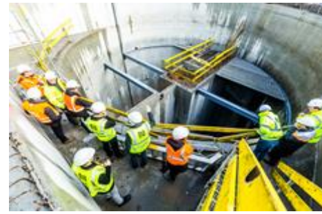
2. Nemo Link Subsea HVDC-interconnection with UK
