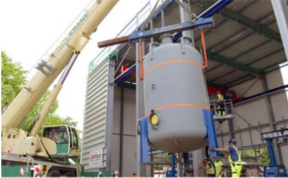
The two large electric boilers for the Power-to-Heat (P2H) project between Hamburger Energiewerke and 50Hertz have been successfully installed. By the end of this year, the P2H system must provide about 27,000 apartments with green city heating. The system converts electricity into heat when plenty of wind energy is available and grid congestion is imminent. 50Hertz is financing the 80 MW plant with €31.5 million.
